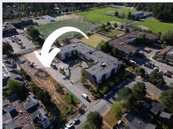
Arial view of construction for KinVillage Phase 1 Independent Living/Enhanced Day Program for Older Adults
